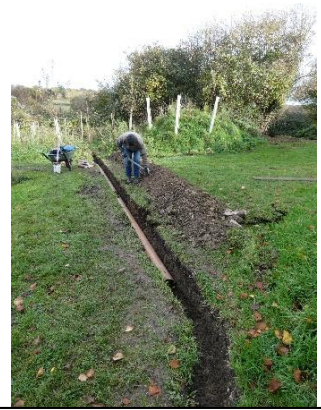
Piped ditch at base of bund
