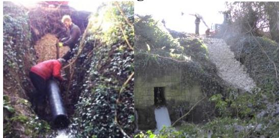
One of our worries has been the erosion under Beechwood Lane, caused by the stream and various springs, which had resulted in a dip in the road and a large hole underneath it. Thanks to help from SDNPA and the work by A D-G Groundworks, the water has been directed through a pipe to join the main stream and the hole has been filled with chalk.
